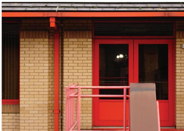
**Figure 54.** Example of poorly located a down-conductor.
