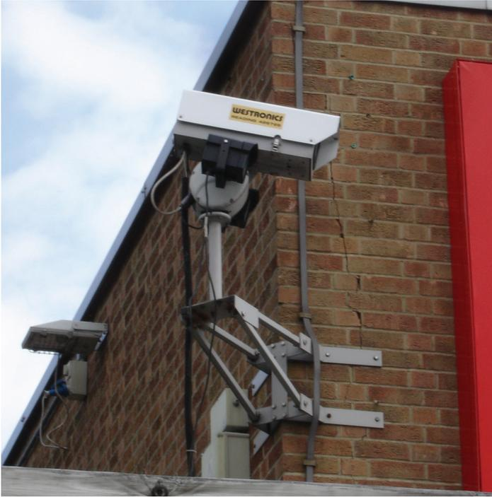
**Figure 15.** Violation of separation distance due to poor design and later additions to structure.
