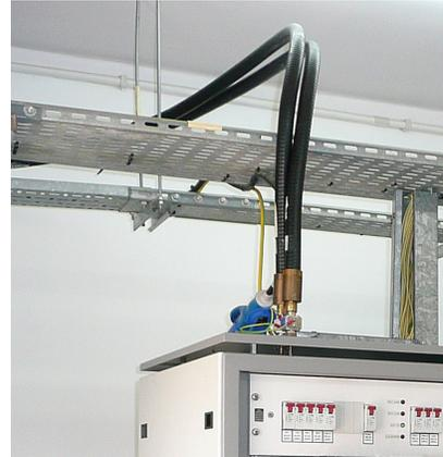
**Figure 113.** Incoming antenna circuits require protection.
